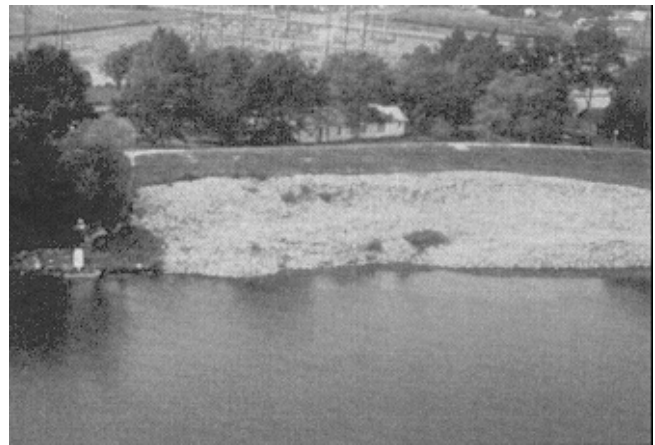
Figure 6-22. Revetment necessitated by encroachment of bank caving on levee
