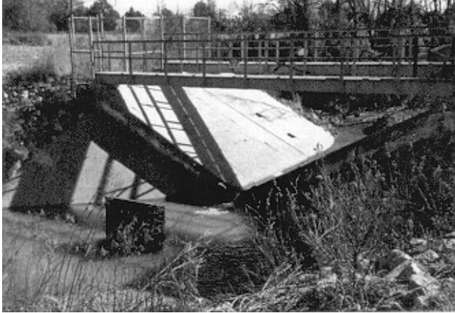
Figure 6-12. Flume-type grade control/gauging structure
