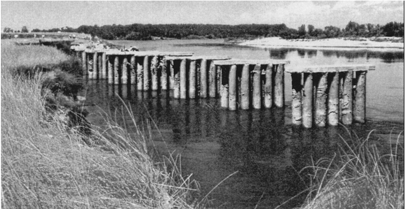
Figure 3-18. Flanking of experimental bank protection on Sacramento River
