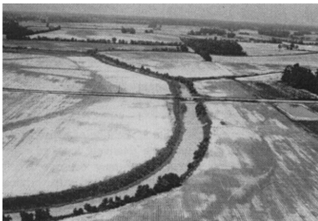
Figure 3-5. Realigned channel without serious instability problems
