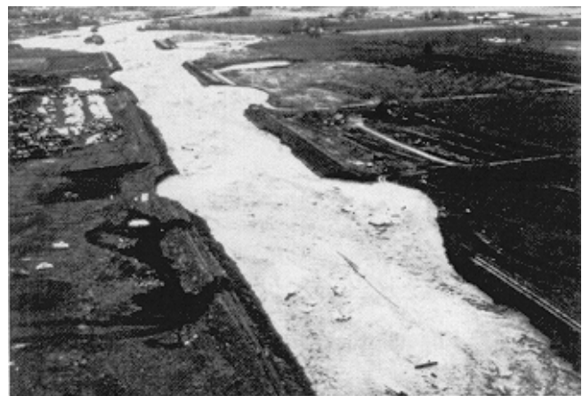
Figure 3-6. Lateral instability in realigned channel
